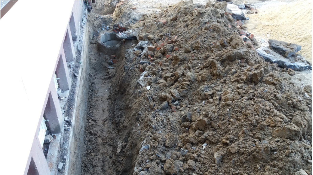
Primary School in Minoga
