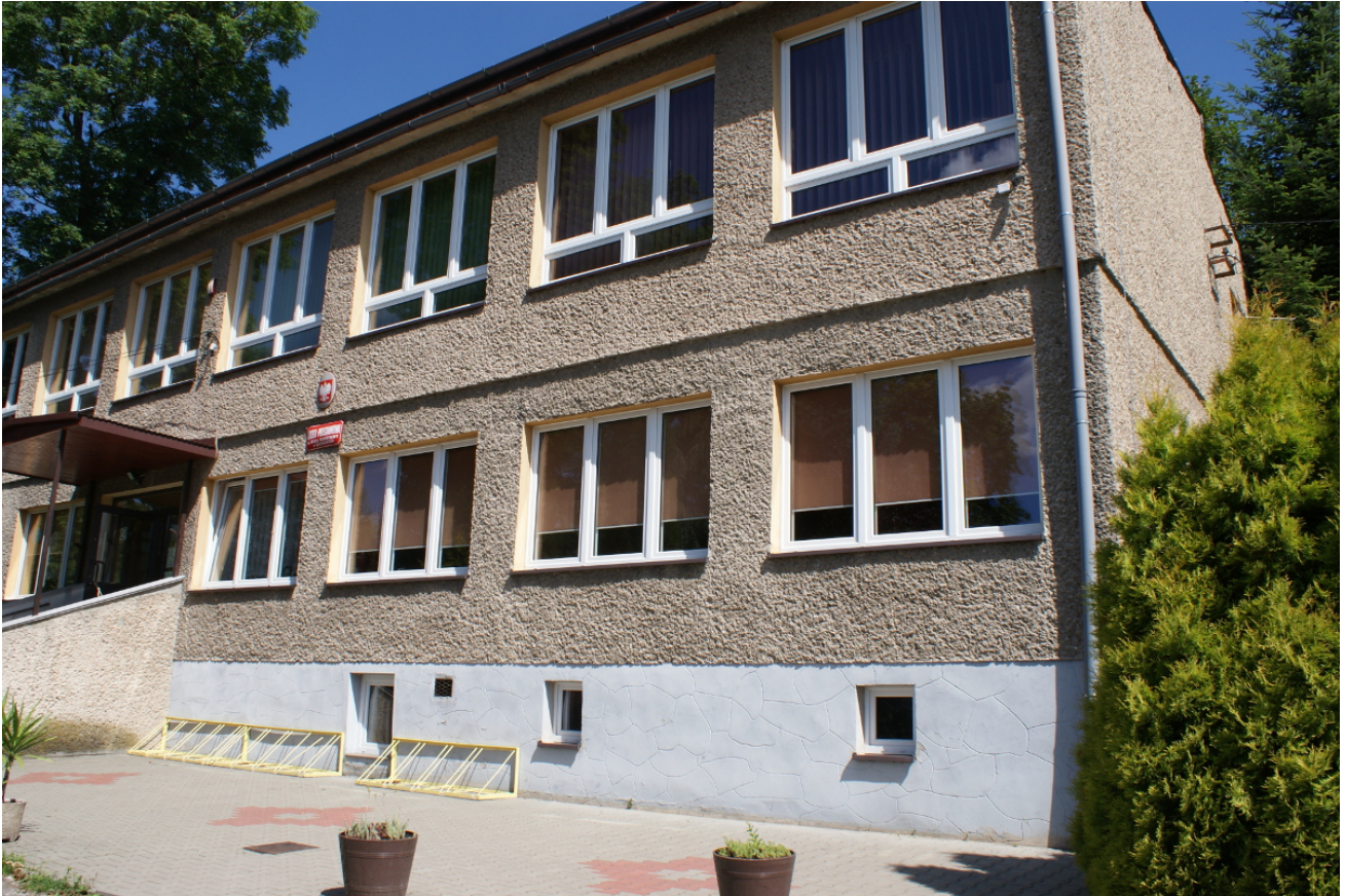
Primary School in Minoga
